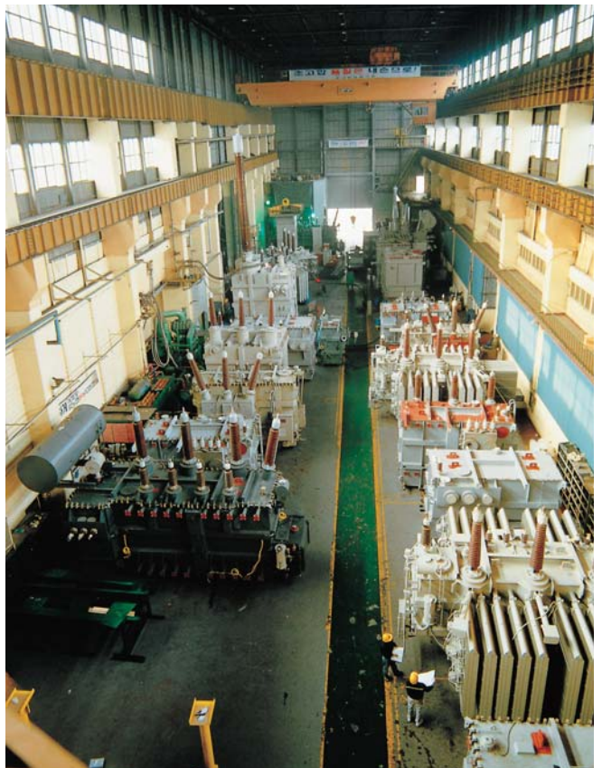
EHV Transformer Assembly Shop
