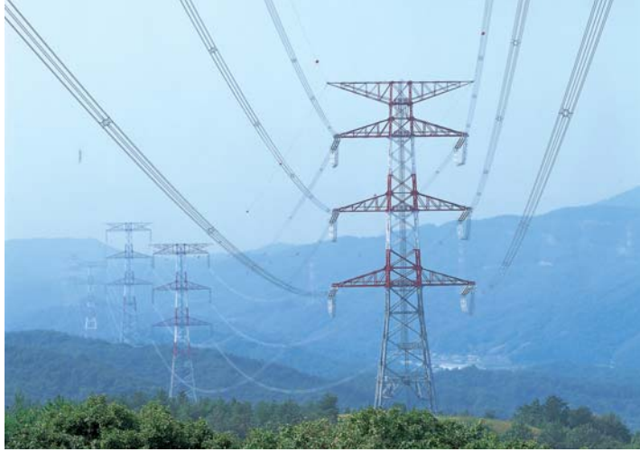
Pipe Tower for 800kV Transmission Line
